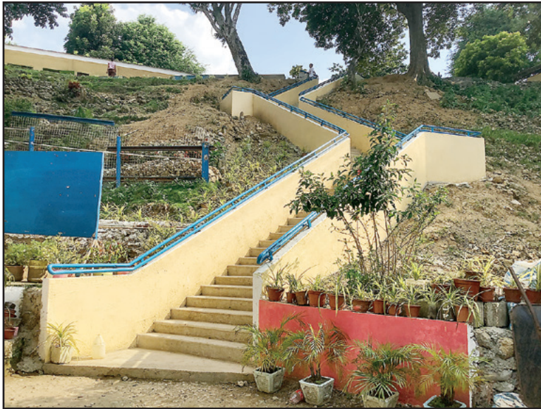
New stairs at LaRosa Elementary School.
